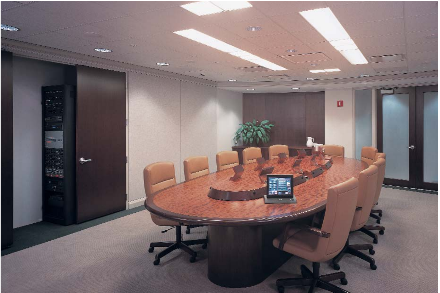
NAR boardroom from front, with videoconference lighting. Note the rack in closet at left; the doors in table open to reveal network and projector connections, and the florescent fixtures in ceiling positioned to put soft lighting on participants' faces.
