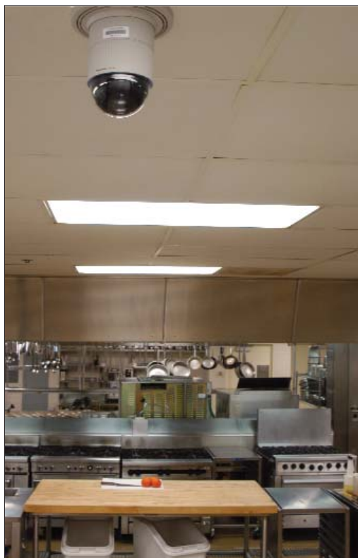
The dome of this high-end Panasonic CCTV camera protects the camera mechanism from airborne grease that's unavoidable in the kitchen.
