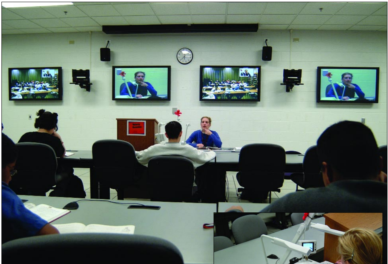
This Latin language class originates at Payton but includes students from Von Steuben High School. The distance learning system includes three robotic cameras, four Pioneer plasma displays and an operator's station with source equipment, codec and controls (shown on cover). Instructors use the document camera in place of a blackboard (see photo at right).
